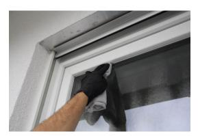
**Step 7: Wiping of the window with polishing cloth**
