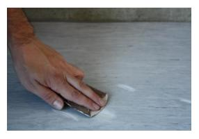
Step 11: Sand the damaged area
